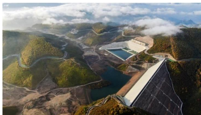
Figura 1 – A Fengning Pumped Storage Power Station. Fonte: State Grid Corp da China
